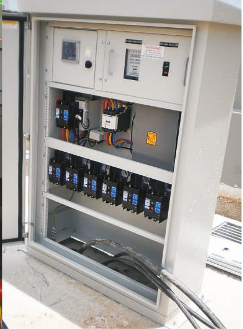
Out-Door Type Feeder Pillar
